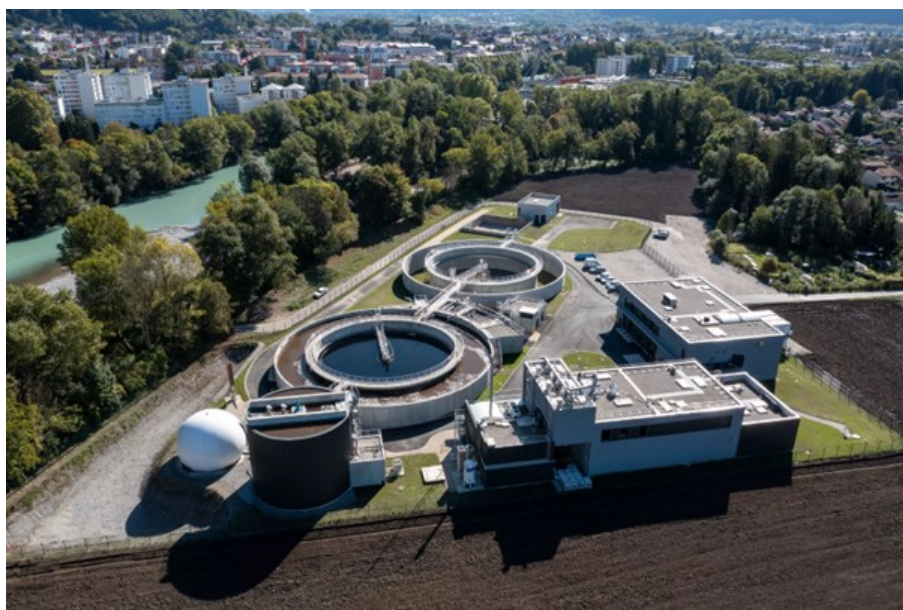
Figure A.2: Aerial Photo of the WWTP of Bonneville (activated sludge)
